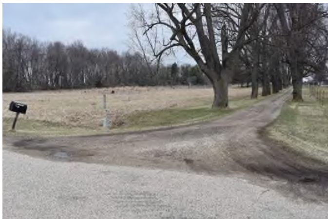
View of the existing and proposed access road facing east from Cumberland Avenue.
